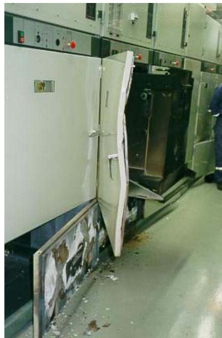
FIGURE 1: A cubicle damaged by arc short-circuit.
